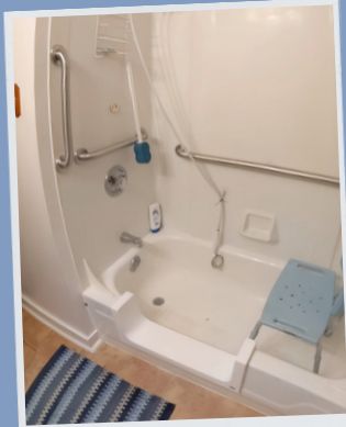
A tub cut-out helps a senior safely step into their shower.
