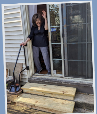
It is much safer for Geraldine to enter and exit her home using a handrail and custom built steps.
